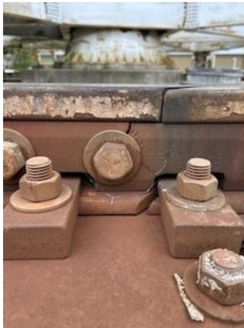
Figure 25: Splice Bar
