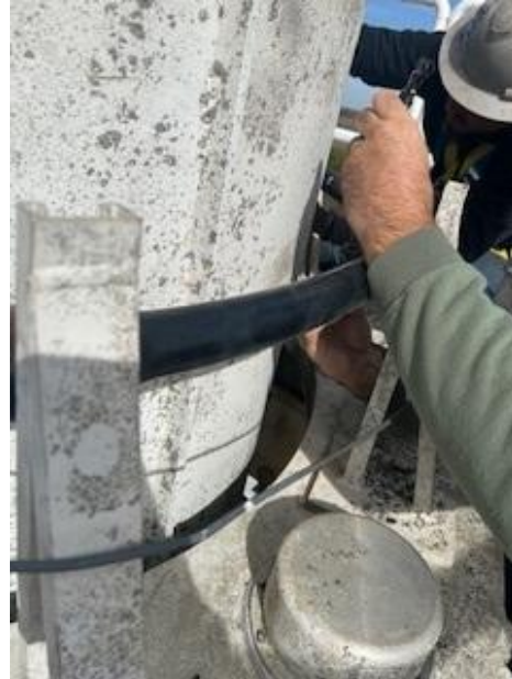
Figure 27: FRM Flex Shaft
