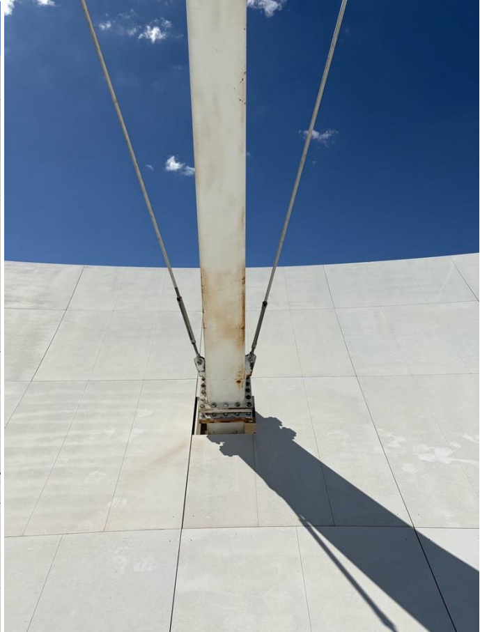
Figure 41: Torsional Rod Assemblies (Guys)
