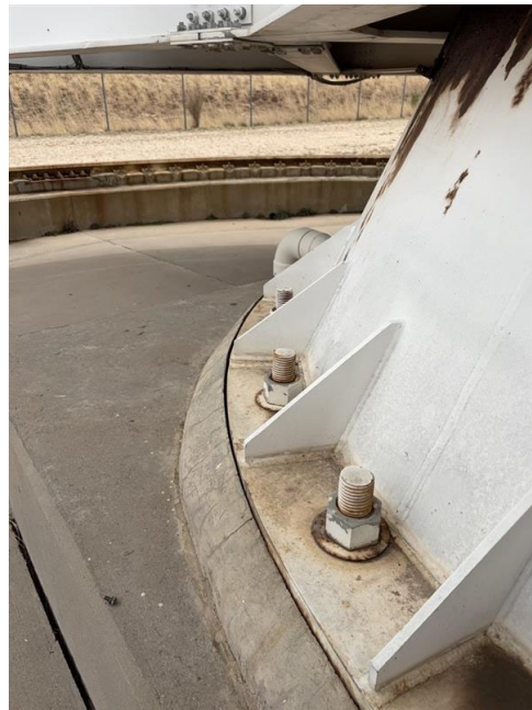
Figure 16: Pintle Bearing Assembly (Exterior)
