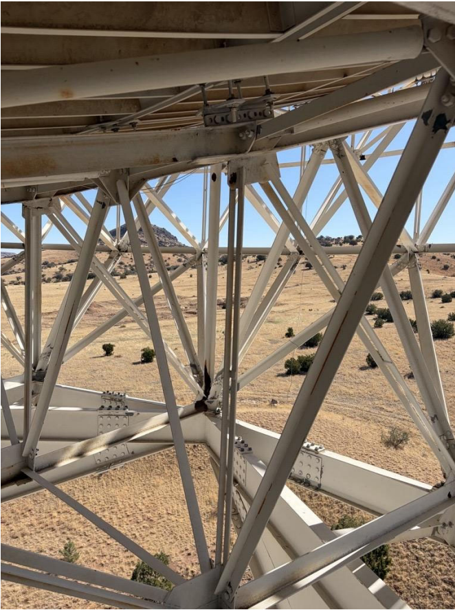
Figure 36: Truss Joint
