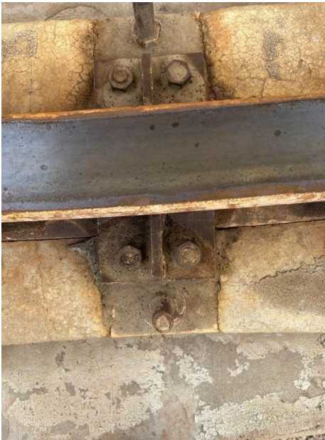
Figure 2: Rail Clips (Bolt No. 70)
