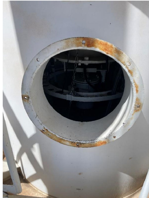
Figure 18: Pintle Bearing Room Port Hole
