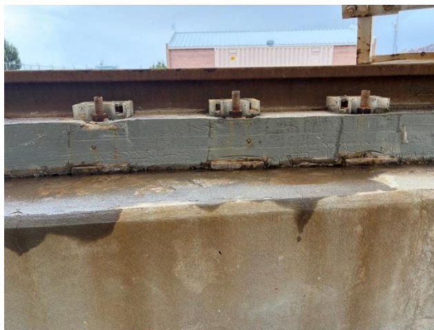
Figure 5: Plates (Bolt No. 3)
