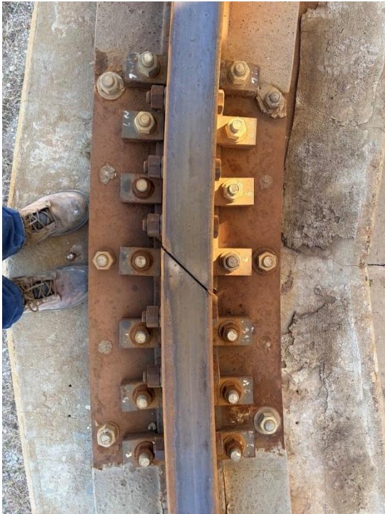
Figure 6: Splice Joint (Bolt No. 41)
