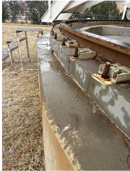
Figure 12: Newly Poured Grout Section
