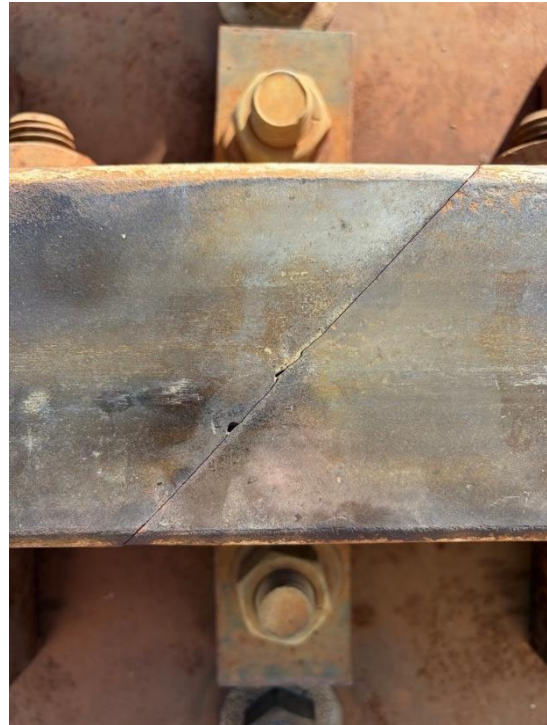
Figure 7: Splice Joint (Bolt No. 61)
