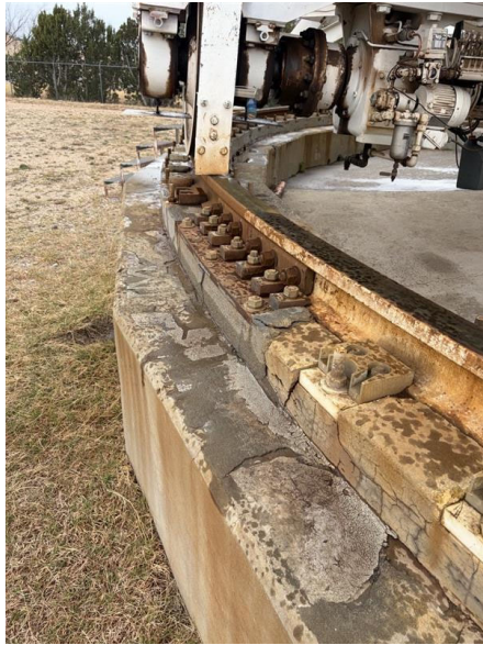
Figure 11: Older Grout Section of Rail
