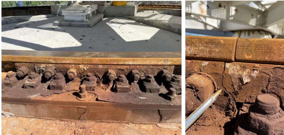
Figure 7: Outer Splice Bar at Bolt #61
