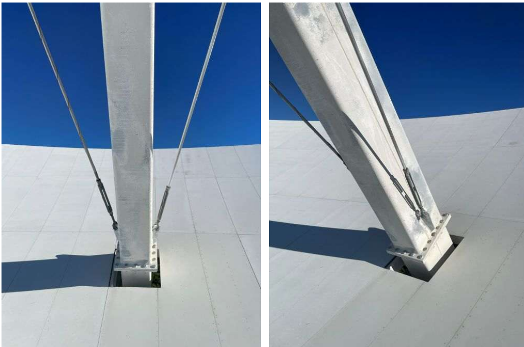
Figure 33: Apex Quad-Leg, Torsion Rod and Guywire 4
