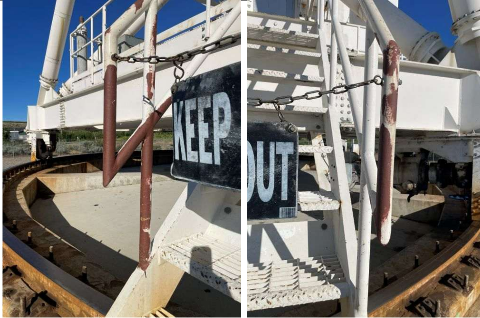
Figure 13: Pedestal Platform - Stairs Handrail
