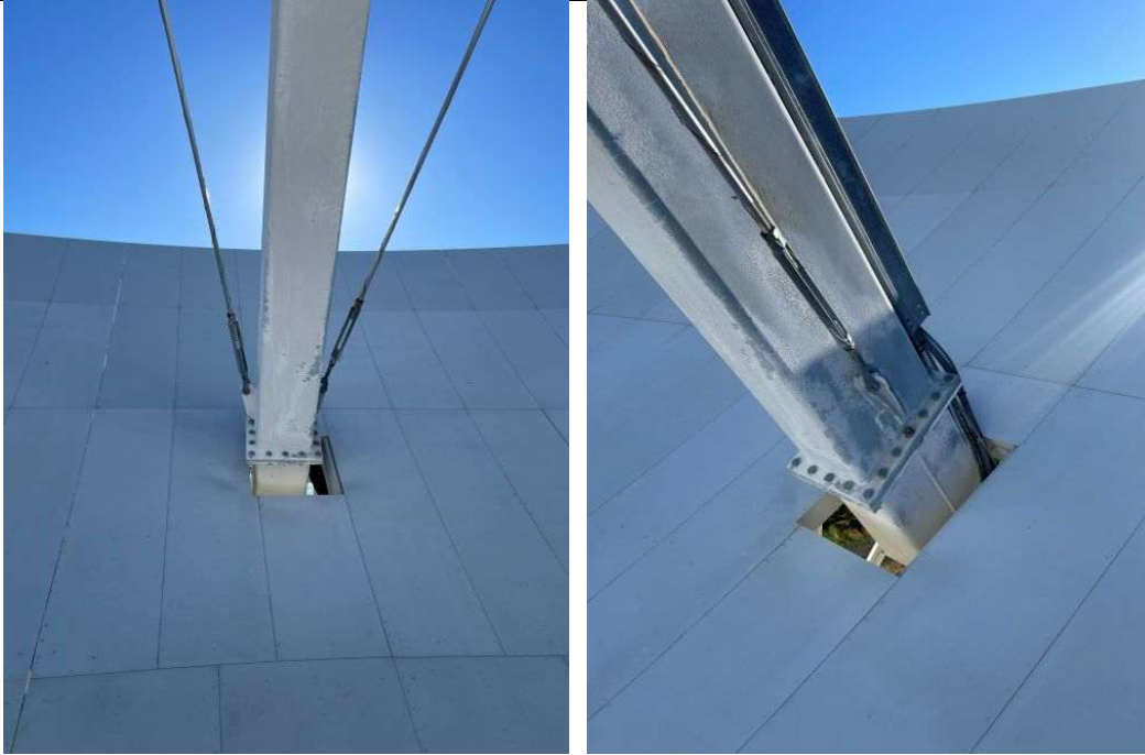
Figure 30: Apex Quad-Leg, Torsion Rod and Guywire 1
