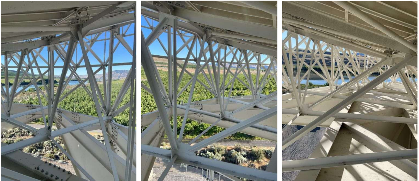
Figure 25: Main-Dish Backup Structure Joints and Beams
