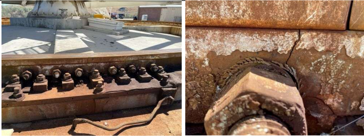
Figure 8: Outer Splice Bar at Bolt #81
