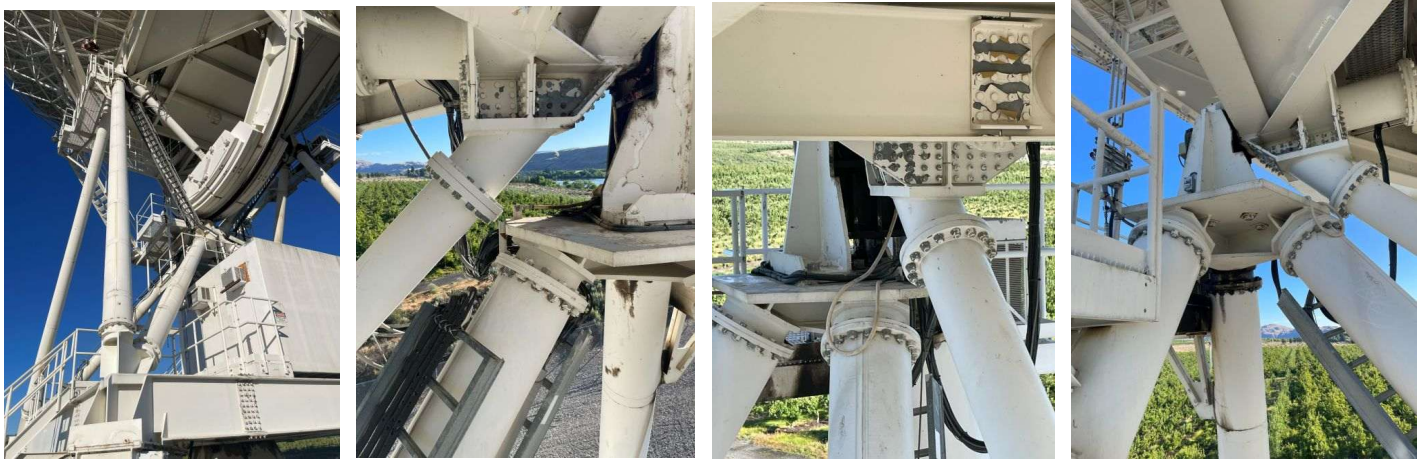
Figure 41: Quadrapod Support and Adjacent Structure
