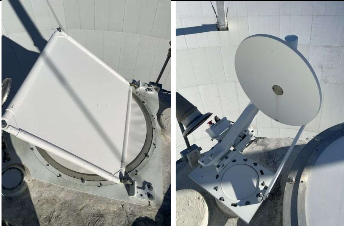
Figure 33: Dichroic Panel and Ellipsoidal Reflector
