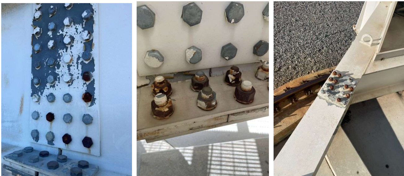
Figure 40: Fasteners on the Lower Structure
