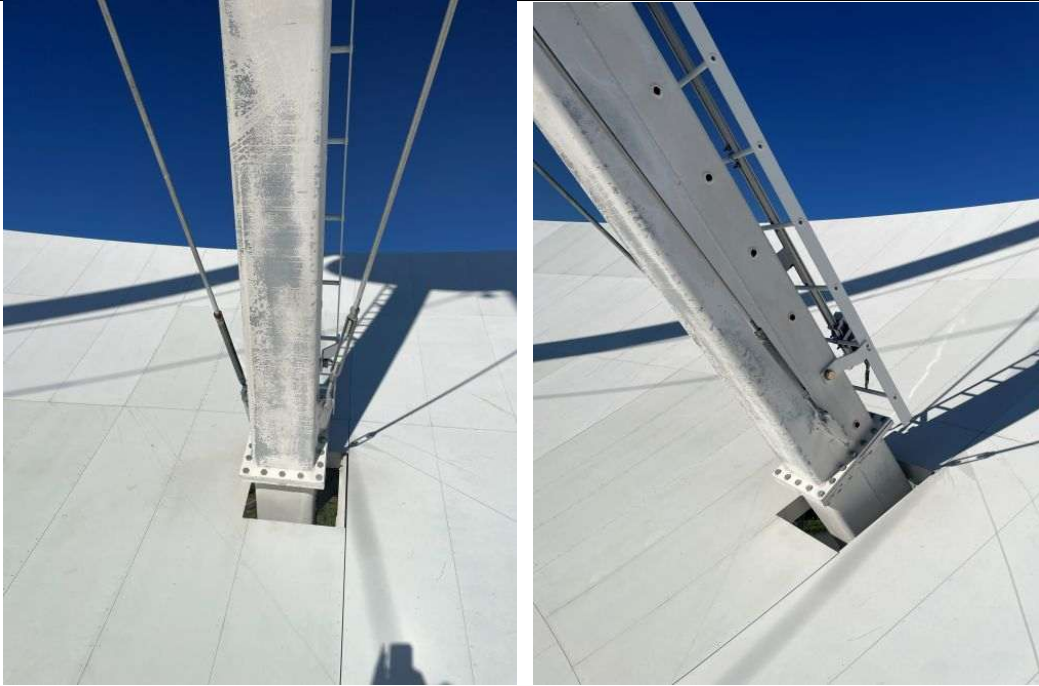
Figure 32: Apex Quad-Leg, Torsion Rod and Guywire 3
