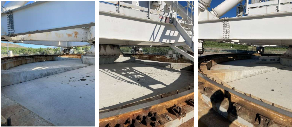
Figure 2: Brewster, WA Concrete Foundation
