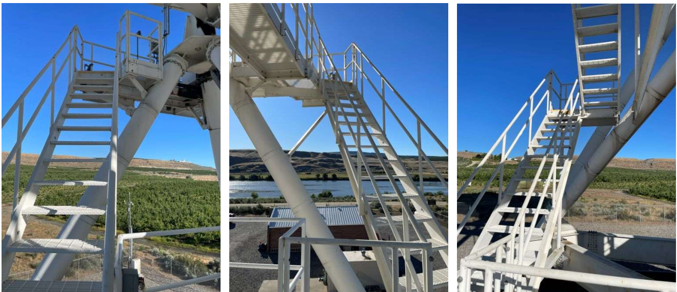
Figure 21: Stairways, Platforms, Gratings, Decks
