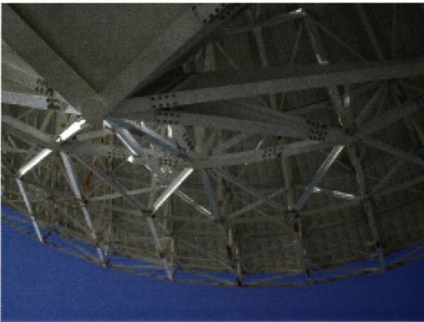
Figure 4: Upper Backup Structure
