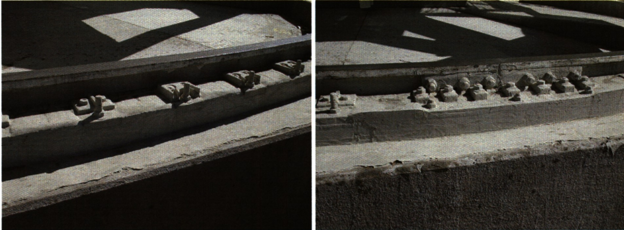
The azimuth rail grout and Vulkem are in excellent condition.
