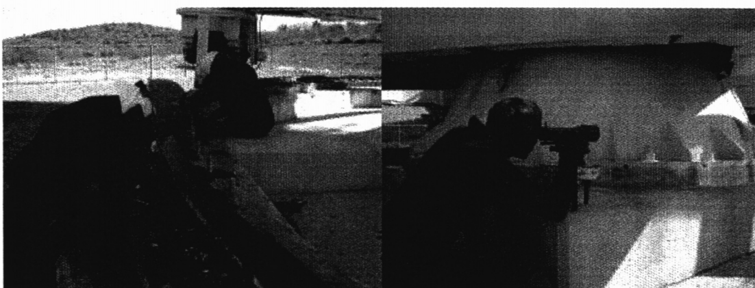
Removing vulkem from the rail.
