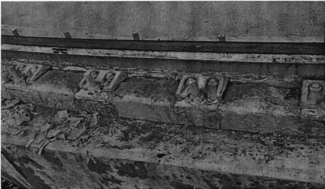
The rail is pulverizing the grout in many spots. Vulchem is deteriorating all over the rail. Site Techs began removing vulchem while the maintenance team was on site and will continue removing vulchem until it is all removed.
