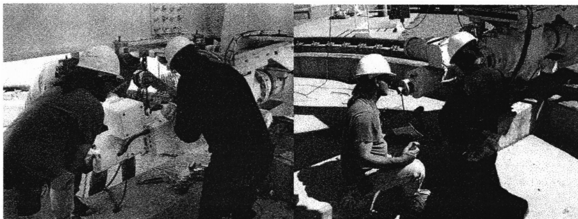
Elevation #2 and azimuth #1 motors were replaced. Digital tachometers were installed and calibrated on the azimuth and elevation motors.
