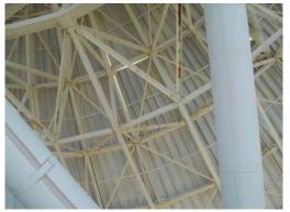
The corrosion on the truss members does not seem to be rapidly progressing even though the paint system has failed as evinced by the above picture.
