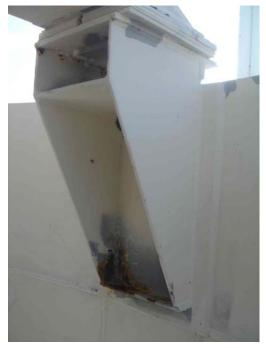
structural brackets used to connect the FRM to the quad legs. This appears to be galvanic corrosion.
