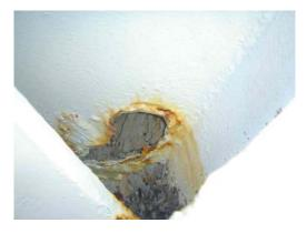
The I-beam inside the antenna "tank", as shown in the next picture is severely corroded. The top of the flange of the Ibeam will need to be reinforced to restore the I-beam to its original strength. There are a few other places on the structure that will also require reinforcement.
