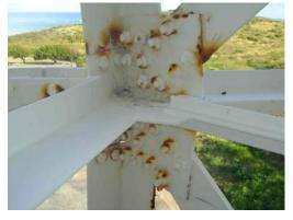
The next picture shows one of the more seriously corroded bolted connections. On this connection, most of the bolt heads have corroded to the point where they will need to be replaced. I estimate that approximately 10% of the backup structure bolts have corroded such that they will need to be replaced.
