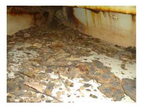
These box sections had severe rust in pockets where water collects. All of the box sections on the antenna will need to be opened, cleaned and painted. Holes should be drilled in the structure to allow water to drain. These drain holes need to have clean edges and then must be properly covered with paint. The drain hole shown below was cut with a torch. Corrosion has severely attacked the hole demonstrating the need for clean painted holes.
