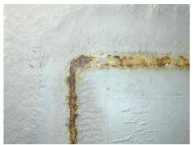
In less than one-year, rust is appearing at the weld on the quad leg patch. This illustrates how the weld material is anodic to the surrounding steel. The silver paint is a product called Rust Bullet that was supposed to eliminate all rust. As you can see, this product is beginning to fail with less than one-year of service. The patches have effectively repaired the damage. However, the paint system on the patches must be repaired or the welded area will rapidly corrode.
