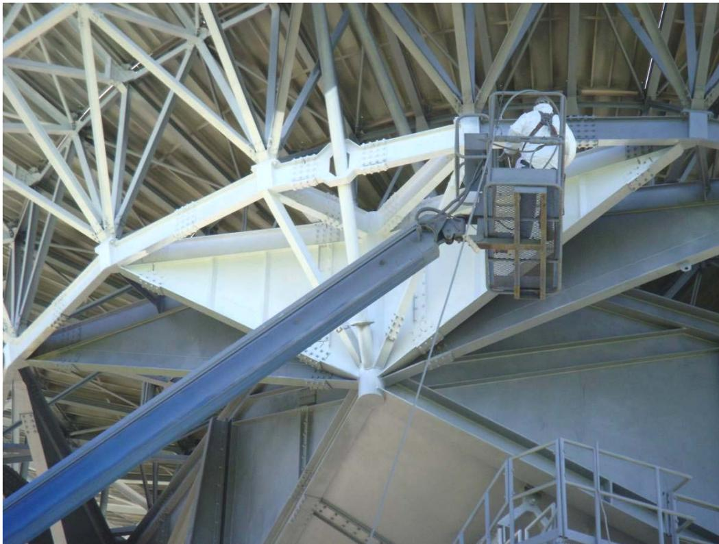
**Figure 1, Applying Topcoat on Structure**
