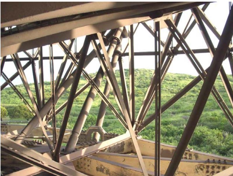
**Figure 7, Backup Structure Truss Primed with Organic Zinc Primer.**
