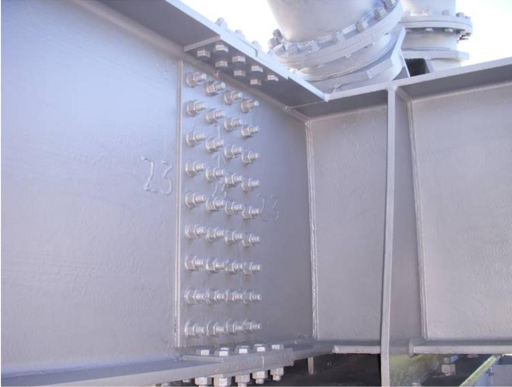
**Figure 9, Epoxy Prime Coat on Remaining Structure.**
