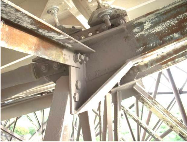
**Figure 6, Stripe Coat Applied by Brush at Connections.**
