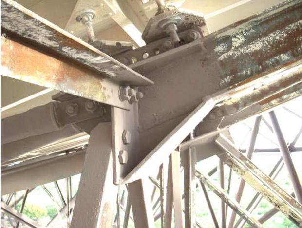
**Figure 6, Stripe Coat Applied by Brush at Connections.**
