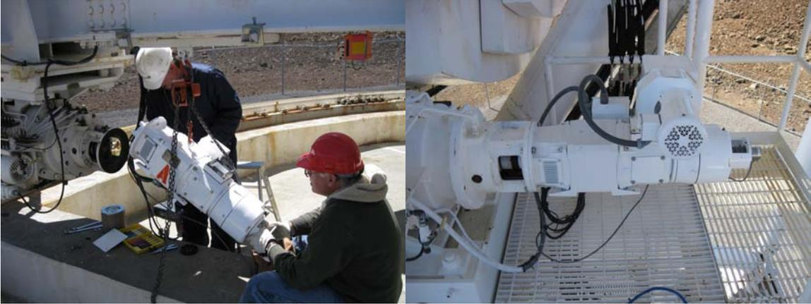
Azimuth #1 motor and Elevation #2 motor were replaced.
