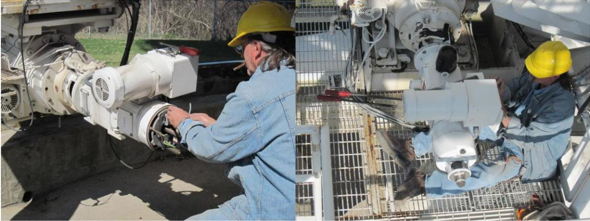
Azimuth motor #1 and Elevation motor #2 were replaced and tested.
