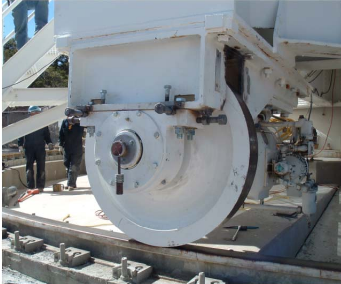
Illustration 1: Wheel During Final Alignment
