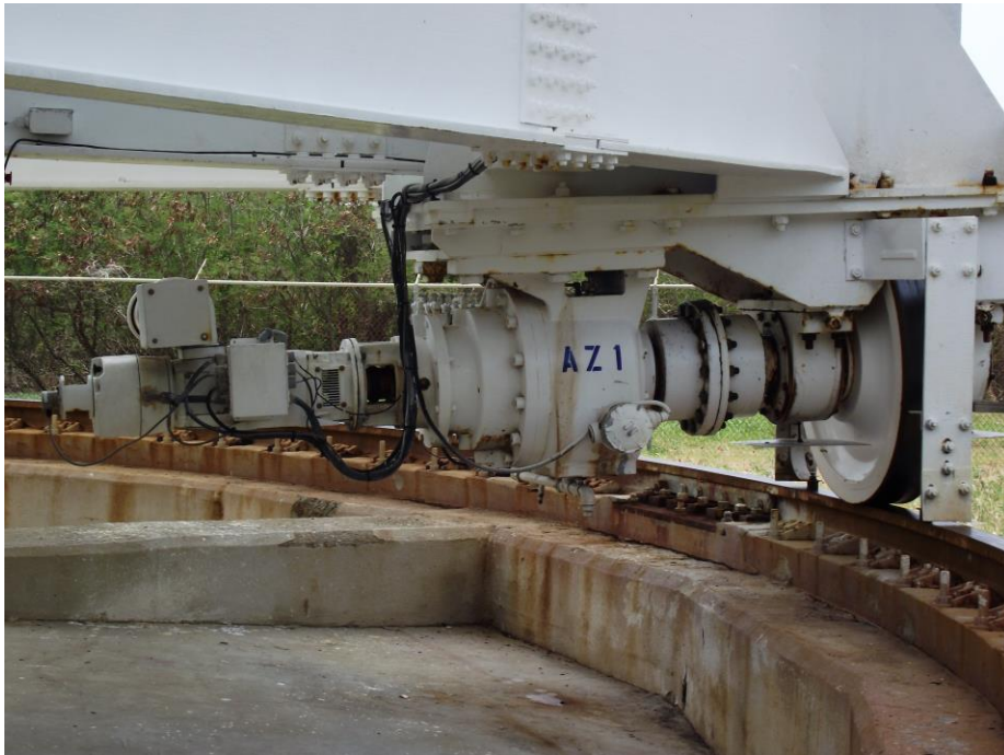
Figure 20, Drive wheel and gearbox assembly corrosion.
