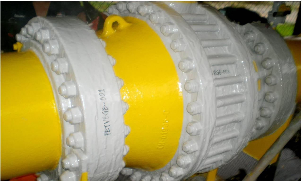
Figure 5: CIST application on complex bolted substrate
