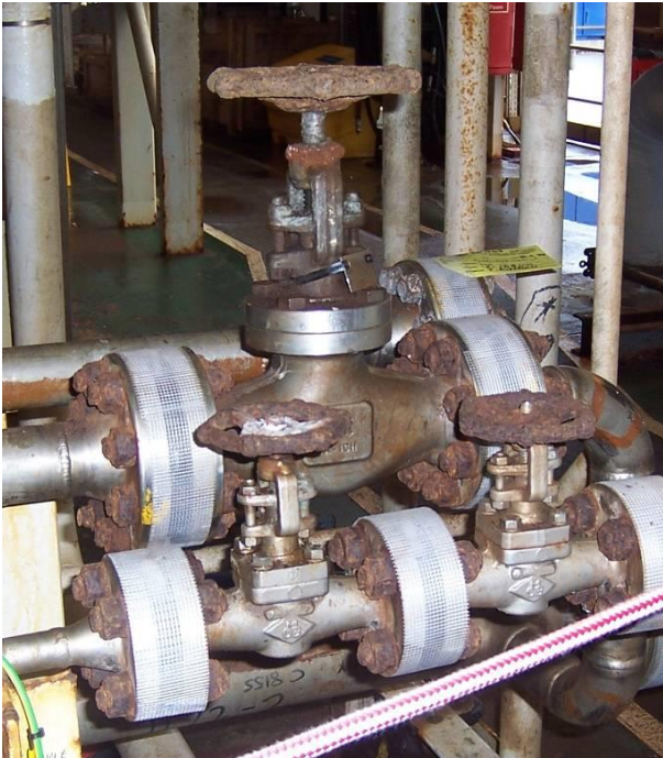
Figure 9: typical substrate prior to application
