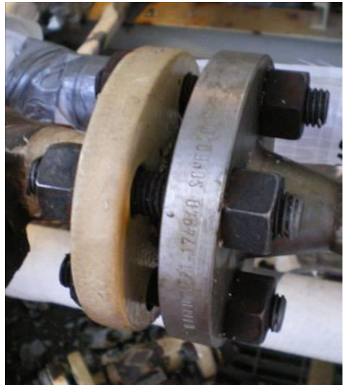
Figure 12: mixed high-alloy and low-alloy fasteners after
