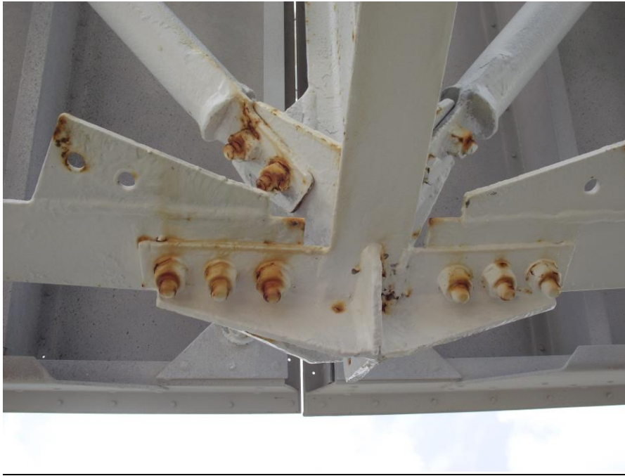
Figure 5, Close up of typical bolted connection.
