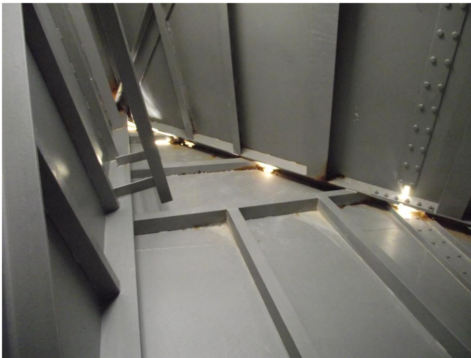
Figure 8, Photograph of the inside of the box structure. This part of the antenna is not subject to UV radiation so it was not painted with the white topcoat.
