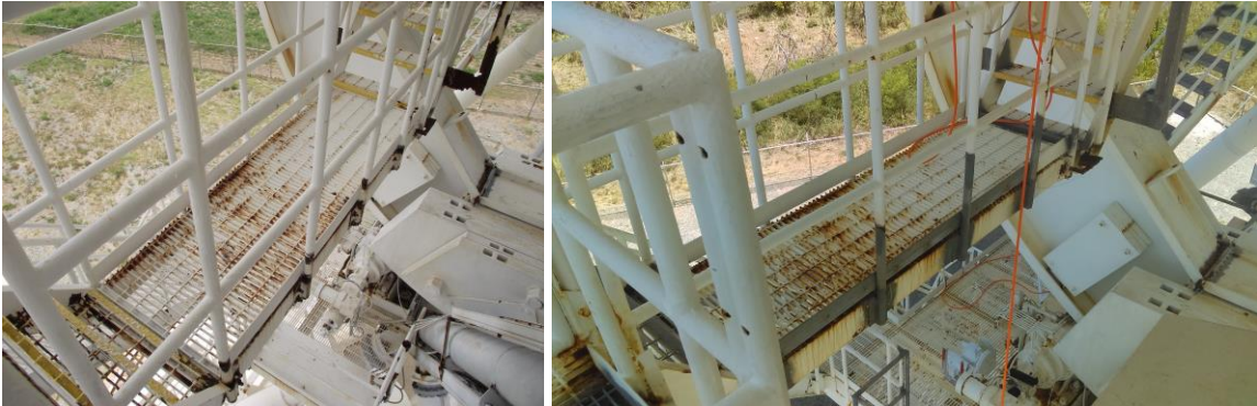
Repair of stair supports and handrail sections.
