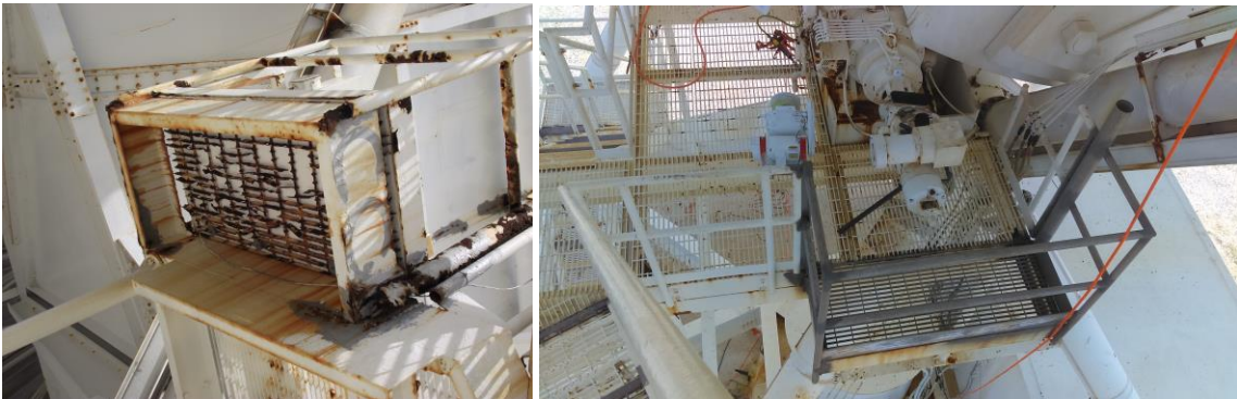
Before and after photos of elevation platform extensions.
