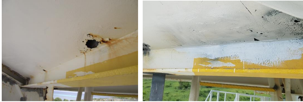
Repaired corroded hole in tank section.
