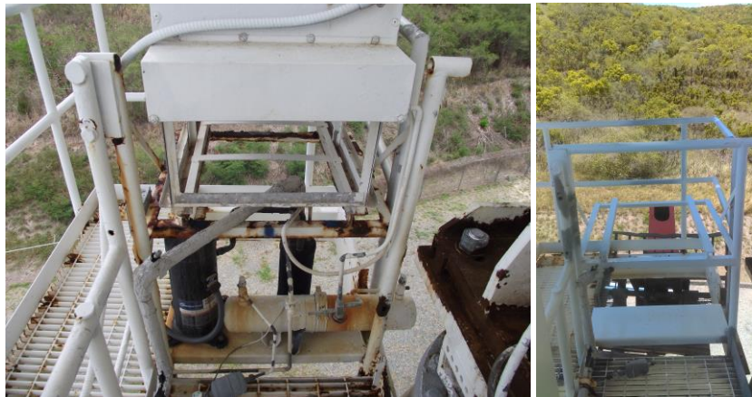
Replaced HVAC platform.
