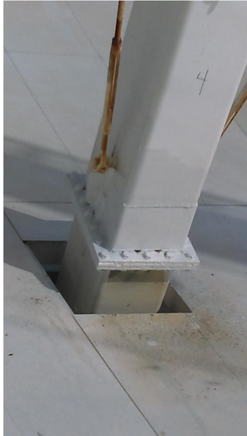
Repaired quad leg with primer and then with epoxy topcoat.
