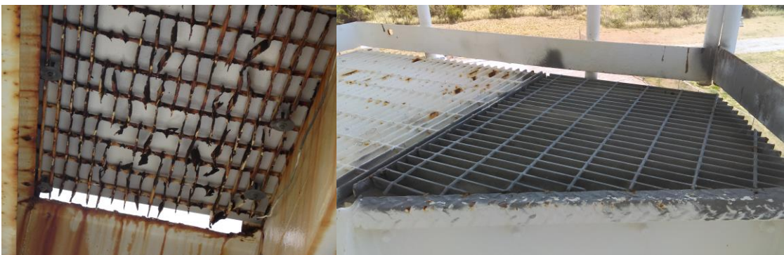
Before and after photos of replaced grating.
