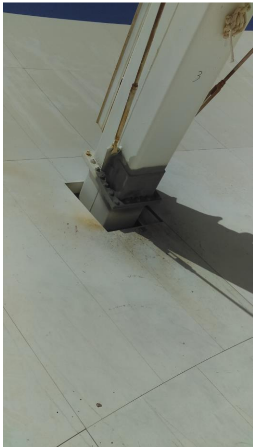
Repaired quad leg with primer and then with epoxy topcoat.
