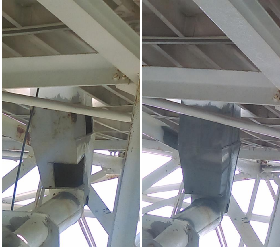
Smaller quad leg patches below the dish.
