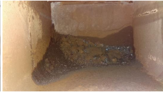
Quad leg with corroded section removed. Accumulated debris inside Quad leg.
