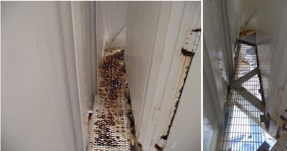
Before and after photos of vertex house grating.
