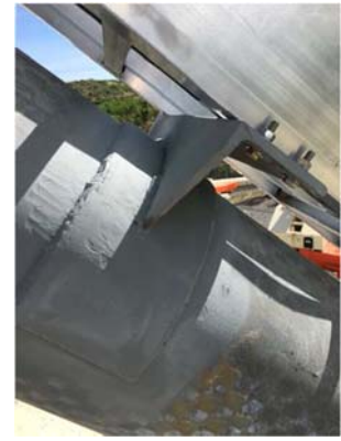
Figure 5: Completed Cable Tray Connection Repair with Cable Tray Installed
