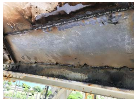
Figure 7: Shear Plate with Weep Holes
