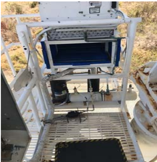
Figure 6: Condenser Platform Pre-Replacement
