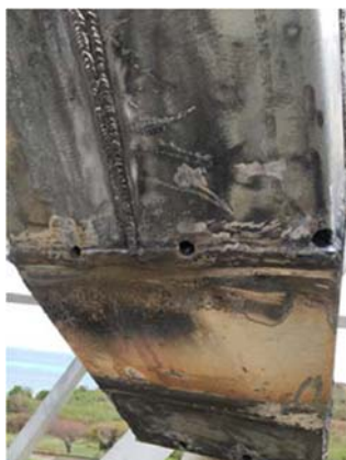
Figure 3: Repaired Quad Leg with Weep Holes
