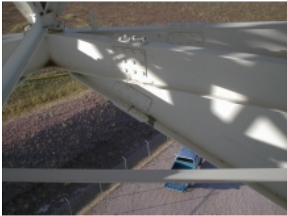
Figure 8: Paint failure
