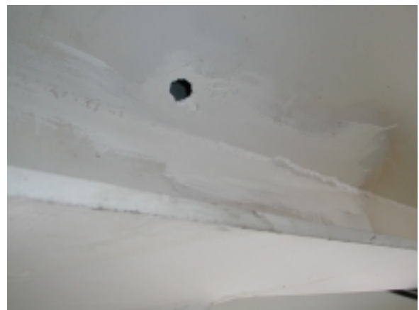
Figure 11: Repaired weld over El bearing
