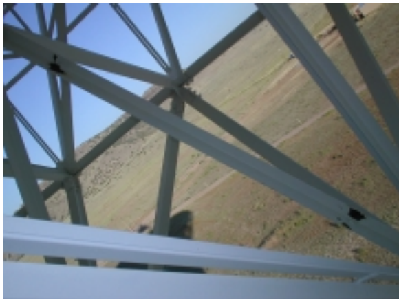
Figure 9: Paint failure
