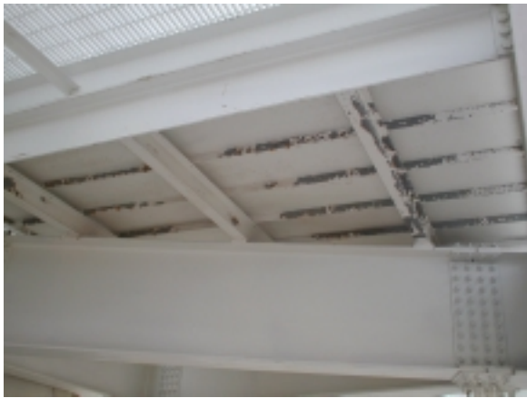
Figure 7: Ped room underside, before scraping
