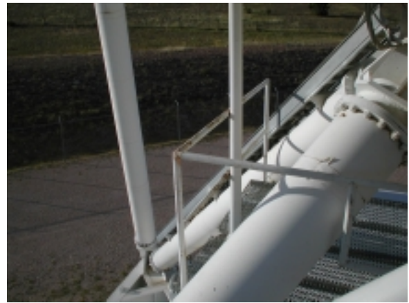
Figure 10: Mid-level handrail before painting
