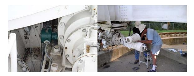
Elevation #1 gear box heater was replaced. New digital tachometers were installed, calibrated and tested on azimuth and elevation motors.
