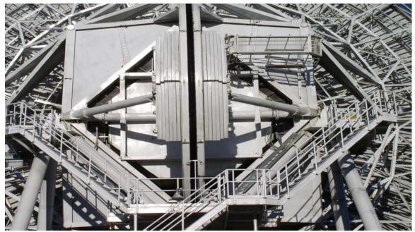
Elevation axle has no visible signs of cracks. Paint is in Fair condition.
