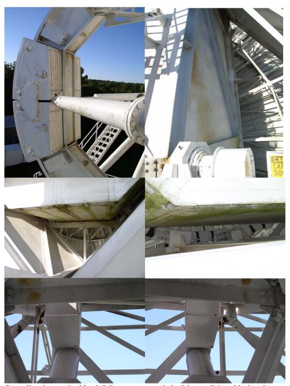
Overall paint on the North Liberty antenna is in fair condition. Notice the drain holes drilled in the quad legs.
