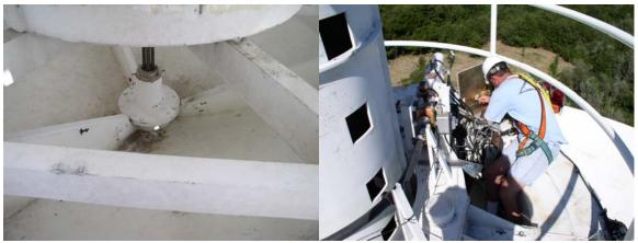
FRM was given a thorough inspection and the focus flex shaft was replaced. Rotation was modified to operate on the West position feedback motor only. The sub reflector did not need rebalancing. The snow tarp was removed and three 1 inch drain holes were drilled in the center on the sub reflector.
