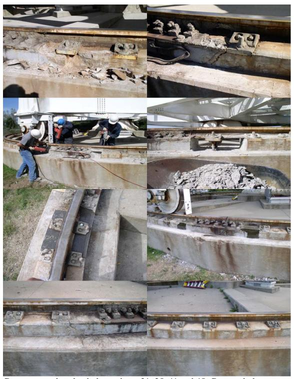
Grout was replaced at bolt numbers, 21, 25, 41 and 45. Grout at bolt numbers, 61 and 65 is degrading. The remaining grout around the rail is in good condition.
