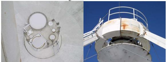
Feed windows & heaters are in good condition. Apex paint is in fair shape.
