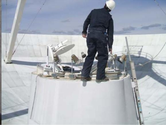
A new dichroic reflector was installed and aligned. The ellipsoid reflector was realigned and is in good operating condition.
