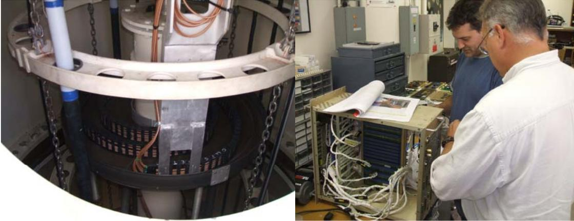
The new IF cable wrap was installed and tested. Four pieces of teflon were added to chaffing power SO cables. The ACU power supply and backplane modification was completed and tested.
