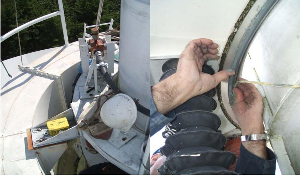
The FRM was given a thorough inspection. The focus flex shaft was replaced along with the INA bearing seal.
