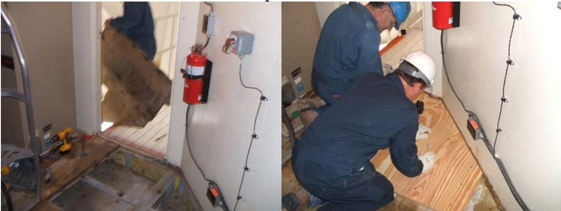
One section of the Vertex room floor was severely damaged by water. This section was cut out and replaced. Vertex room floor tiles were removed for the site techs to seal and paint the floor.
