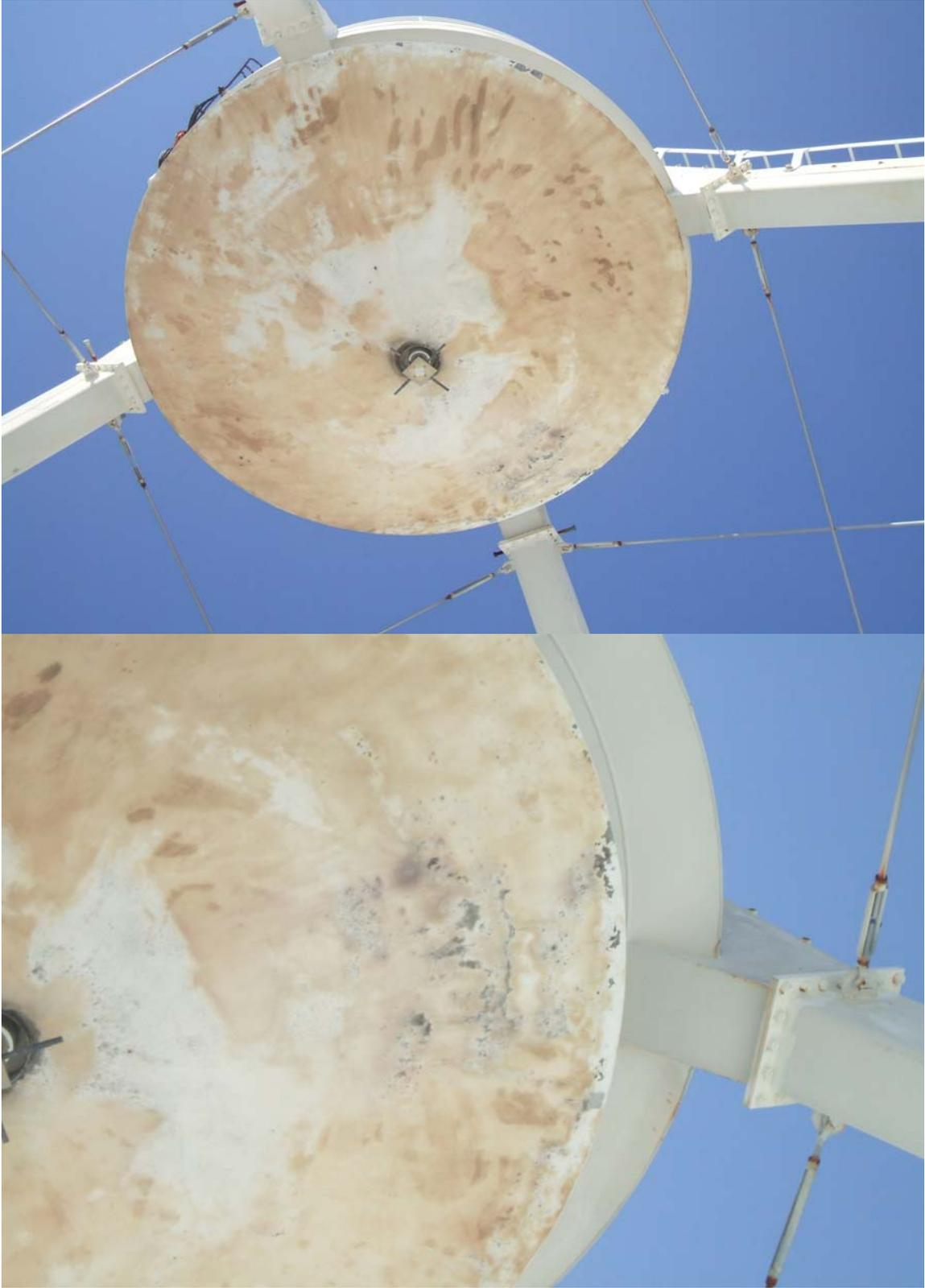
Hancock's sub reflector paint is degrading.
