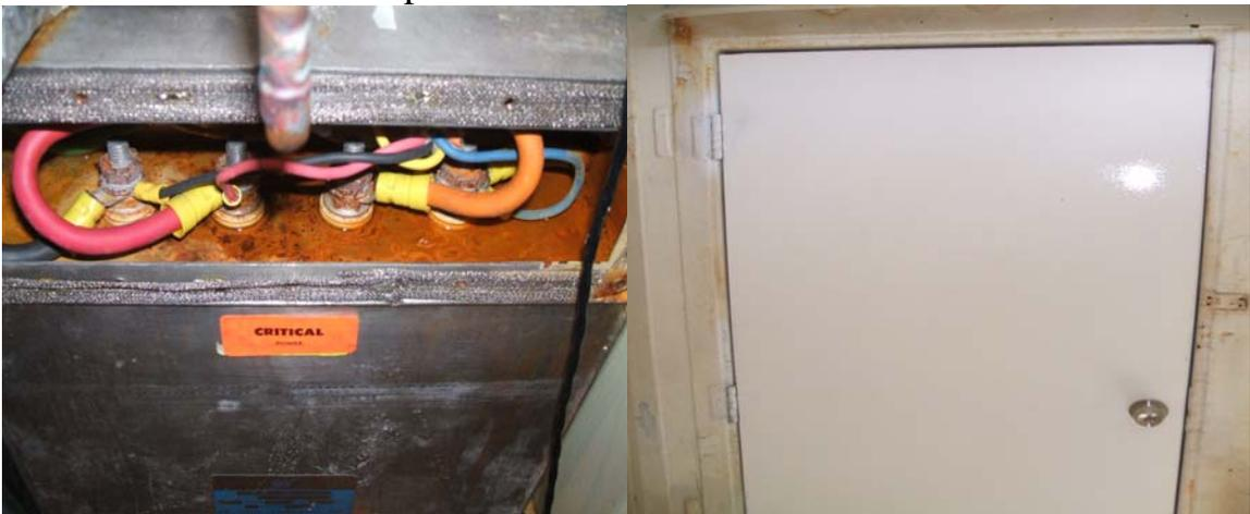
The Vertex room RFI critical power filter was full of water. Vertex room power was shut off. The filter was dried out and connections cleaned. RFI filter leak was located and sealed. The vertex room door was also replaced.
