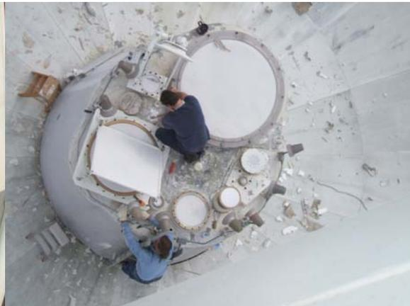
The Elevation synchro side cable wrap was repaired. Vulchem was retaining water on top of the feed cone. The vulchem had to be scrapped off and the feed cone sealed and painted.
