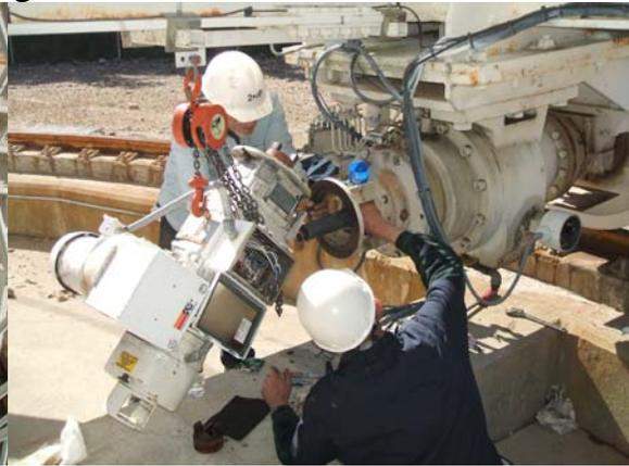
Elevation motors #1 and #2 were replaced. AZ #1 motor needed a new brake assembly. A new blower motor and air box was installed on AZ #2. AZ#2 gear box seal was also replaced.
