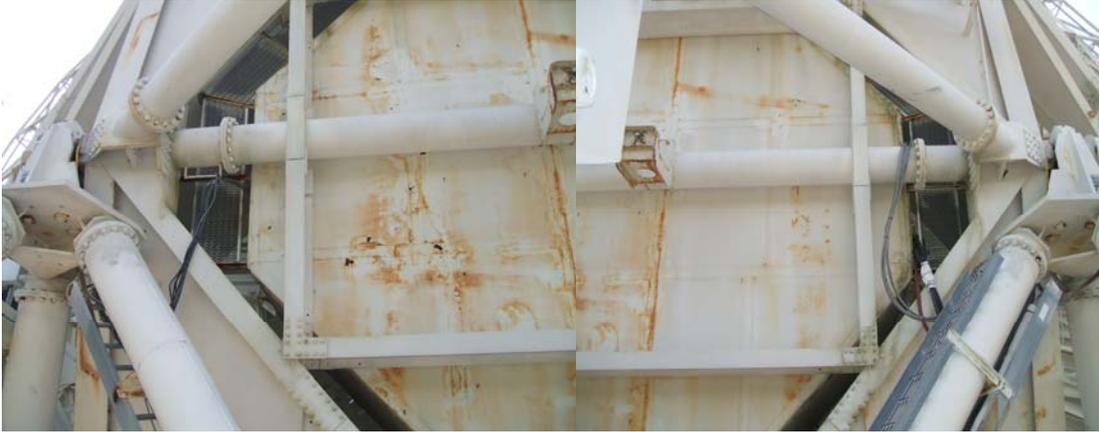
Elevation axle has no visible signs of cracks. Both elevation axle ground cables were replaced. Paint is in poor condition.
