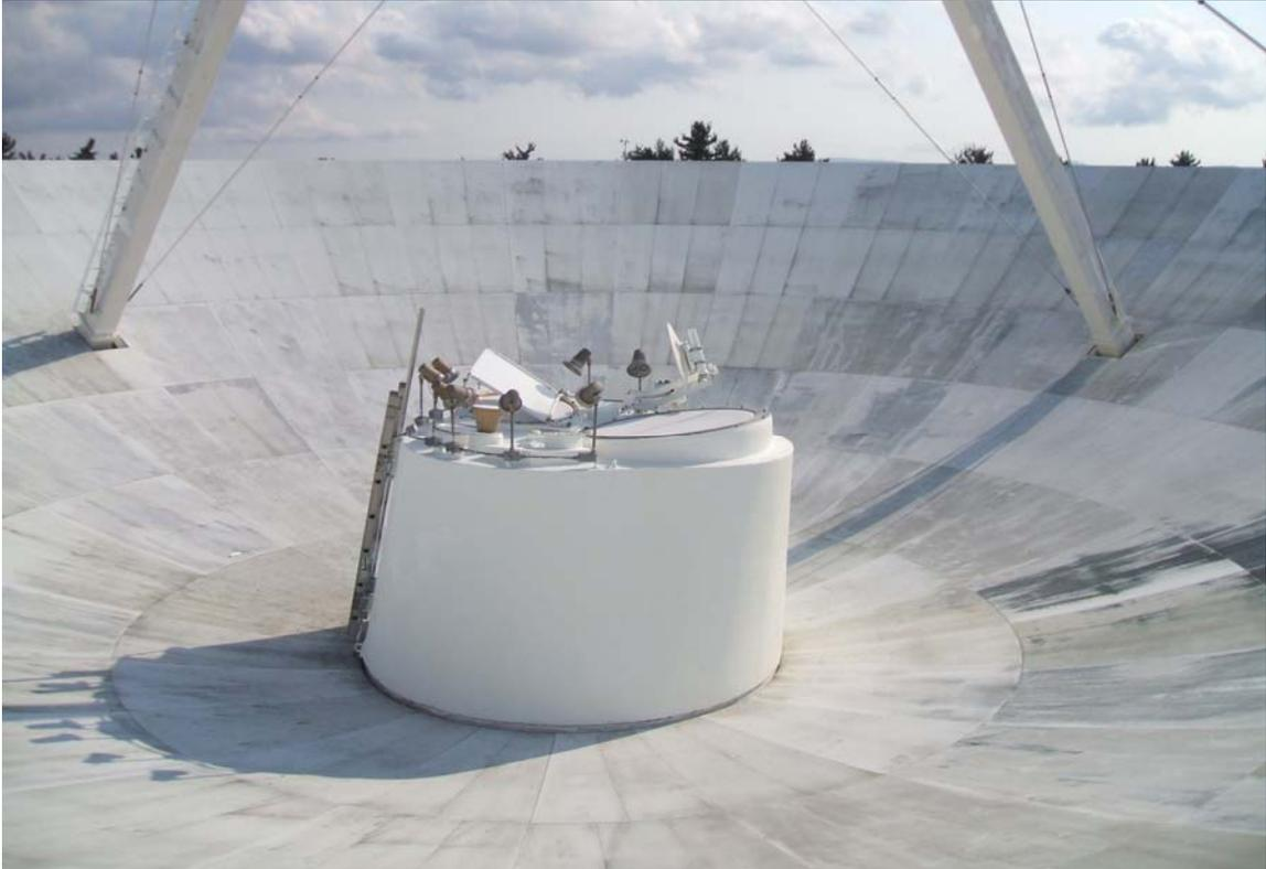
Dish panels are in good condition with no dents. The feed cone was sealed and painted with elastomeric.
