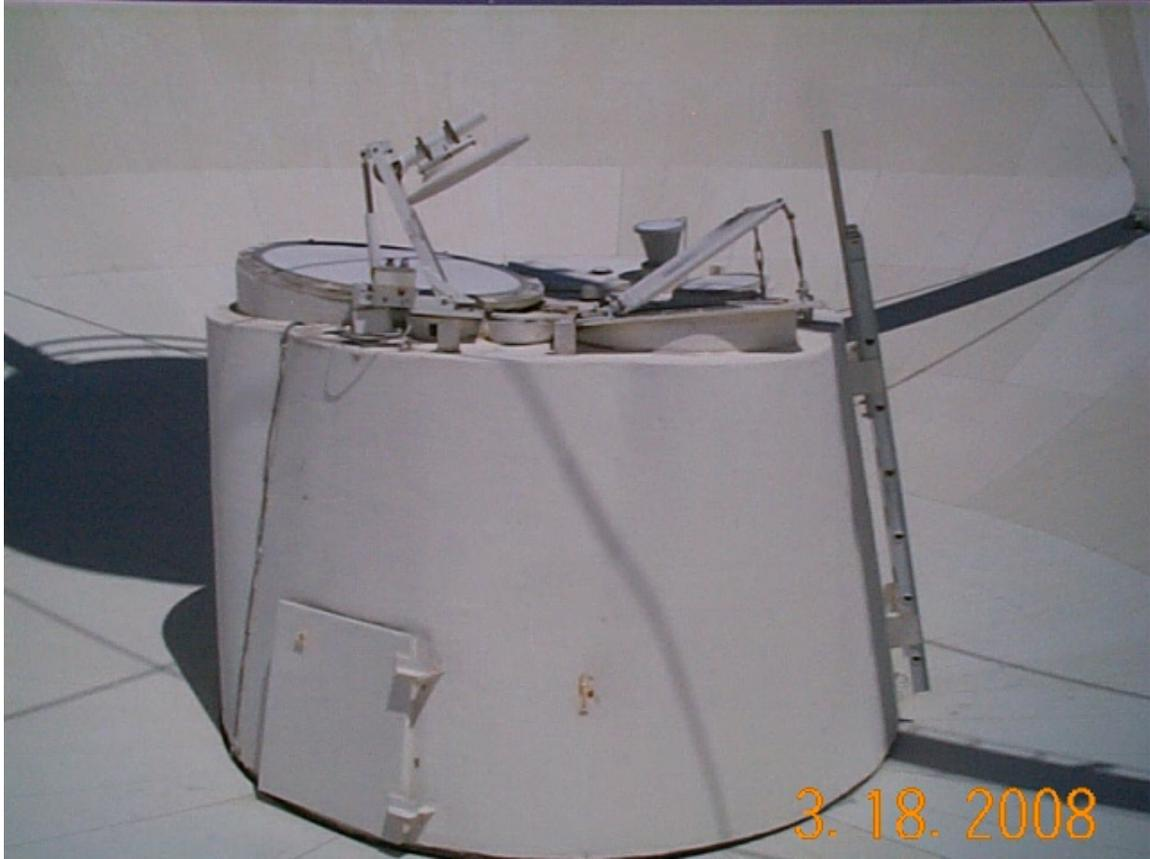
Dish panels are in good condition. The feed cone's elastomeric paint is holding up well.
