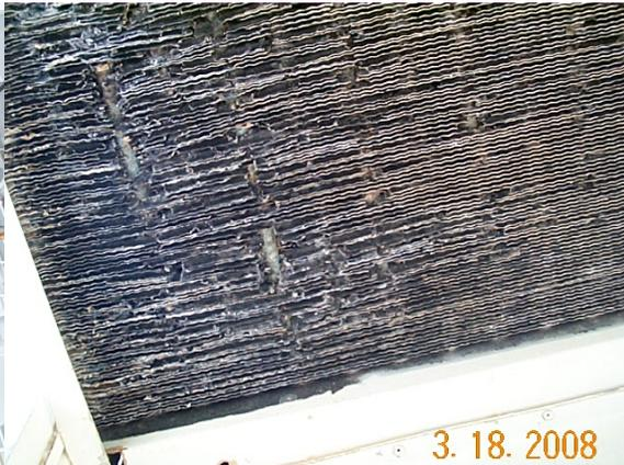
Both CRYO compressors were inspected and are in good condition. Both Contempo condenser coils are deteriorating and will need replaced.
