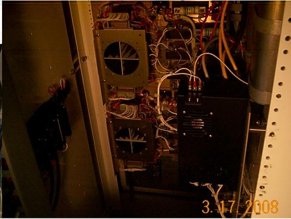
The new IF Cable Wrap was installed and tested. The Site Techs had to install the new drive cabinet power supply shortly before the maintenance team visit due to a failure.
