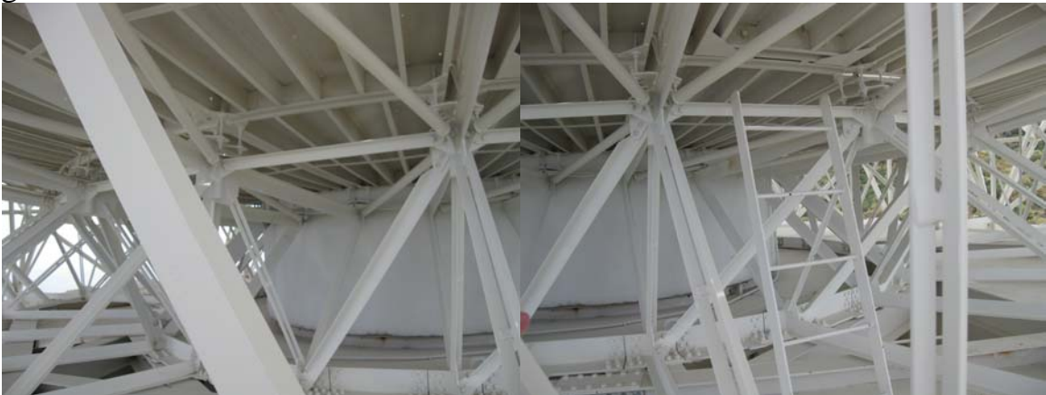
Antenna backup structure is in good condition. Paint is in good condition.
