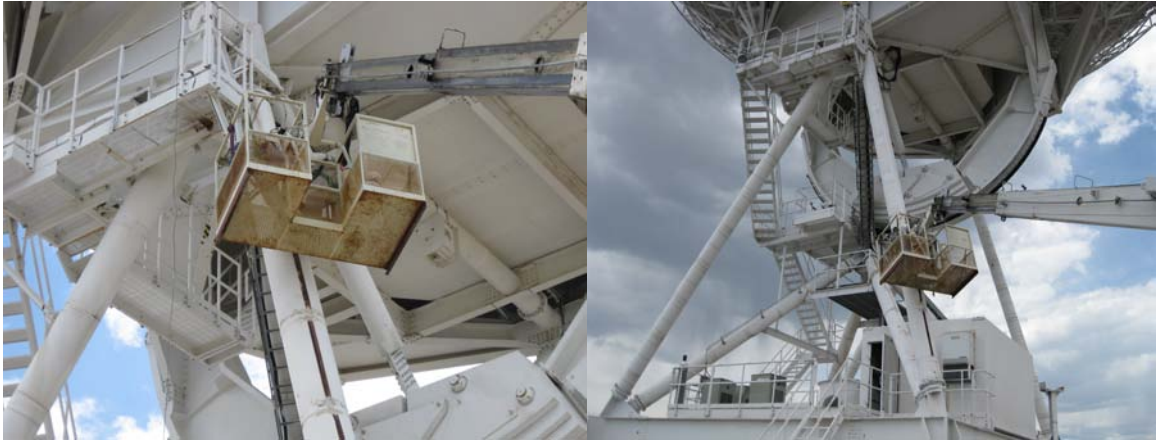
The antenna leg insulation was reattached and banded in several locations.
