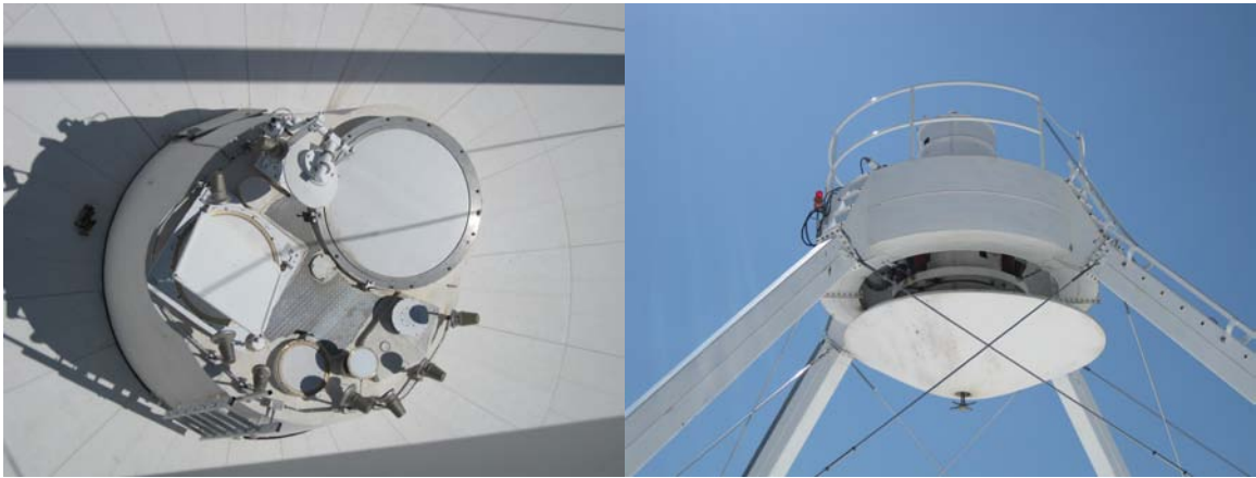
The feed heaters and FE windows are in good condition. Apex paint is in good condition.
