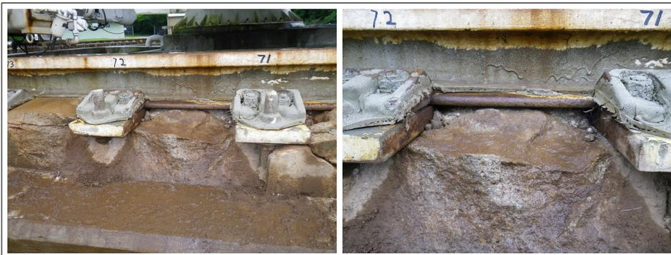
Figure 3: Bolt 72 area before repair
