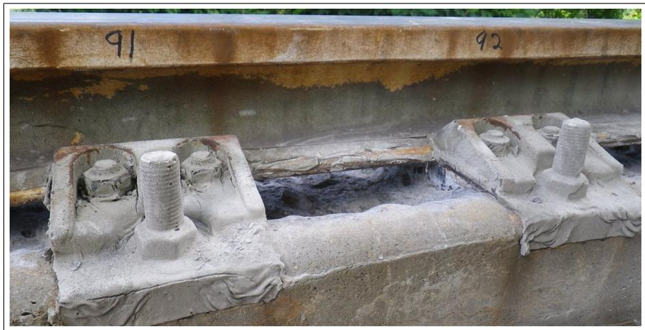
Figure 6: Bolt 91 after grout removal
