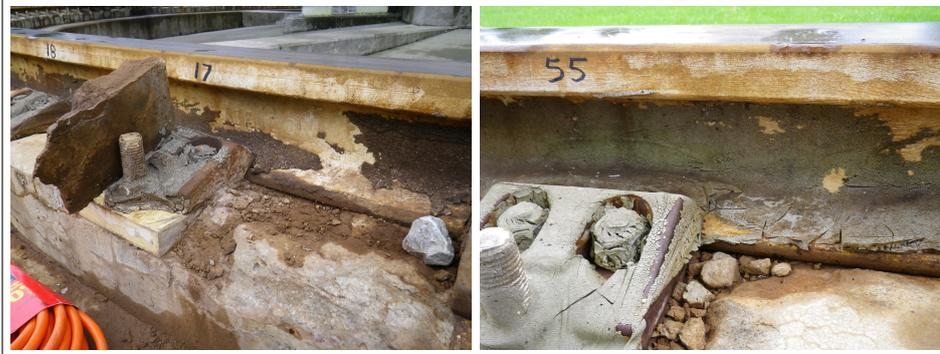
Figure 2: Bolts 17 and 55 before repair
