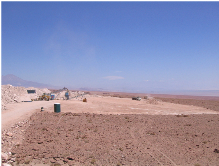
Figure 4: Crushing operations to produce fill material have started. Fill area marked.
