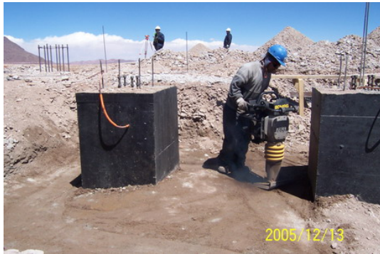
Finished foundation and soil compaction;
