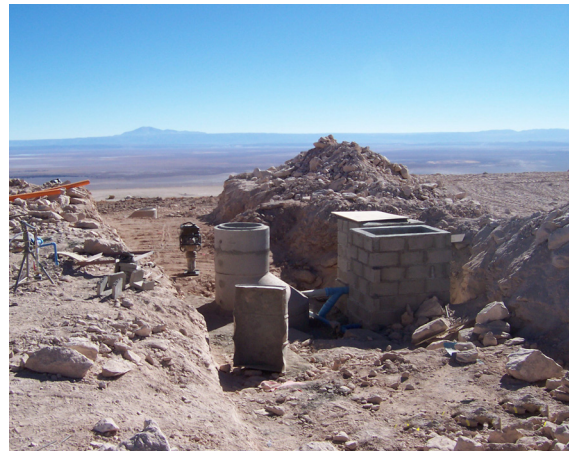
Utilities (water, sewage, electric and FO conduits) for Vertex/Melco/AEM antenna contractors SEF areas.
