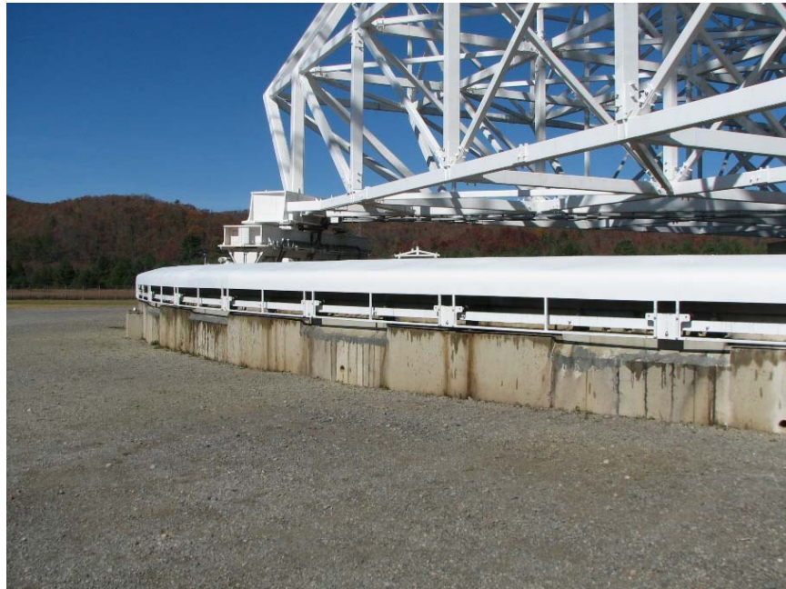
Figure 3. New GBT Azimuth Track covers.
